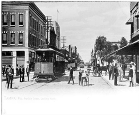
Franklin Street, Tampa, FL
